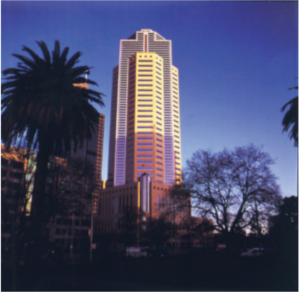
Casselden Place, Melbourne, Australia
